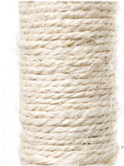
.Timber Pile wrapped with Sisal.
